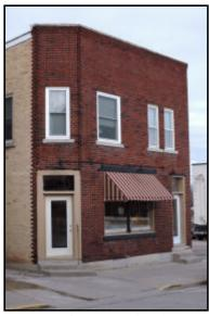
structure. After purchasing the property, Main Street organized a group of volunteers to assist with cleaning out the interior. Nine 30-yard dumpsters were needed to haul away the debris removed from the building. Renovation included removing drop ceilings, patrician walls, subfloors and the rear addition. The original
